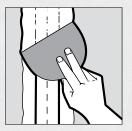
While embedding the tape, remove excess drywall compound from edge and apply as a thin coat over the tape.
